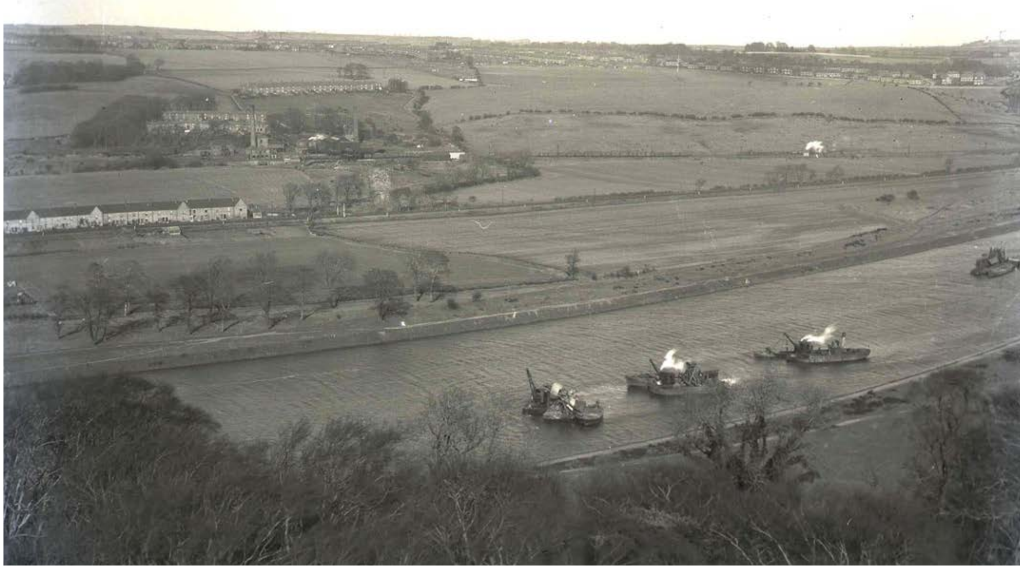
Blayney Row and Throckley Colliery: This photograph was taken around 1900 from the spire of Holy Cross Church in Ryton, looking out across the Tyne to the area just west of Newburn. A line of steam-powered dredgers can be seen at work deepening the channel of the river on behalf of the Tyne Improvement Commission. On the north bank is Blayney Row, built in 1889 for employees of Heddon Brickworks by its owner Cadwallader John Bates of Heddon Hall, and sold to the Throckley Coal
