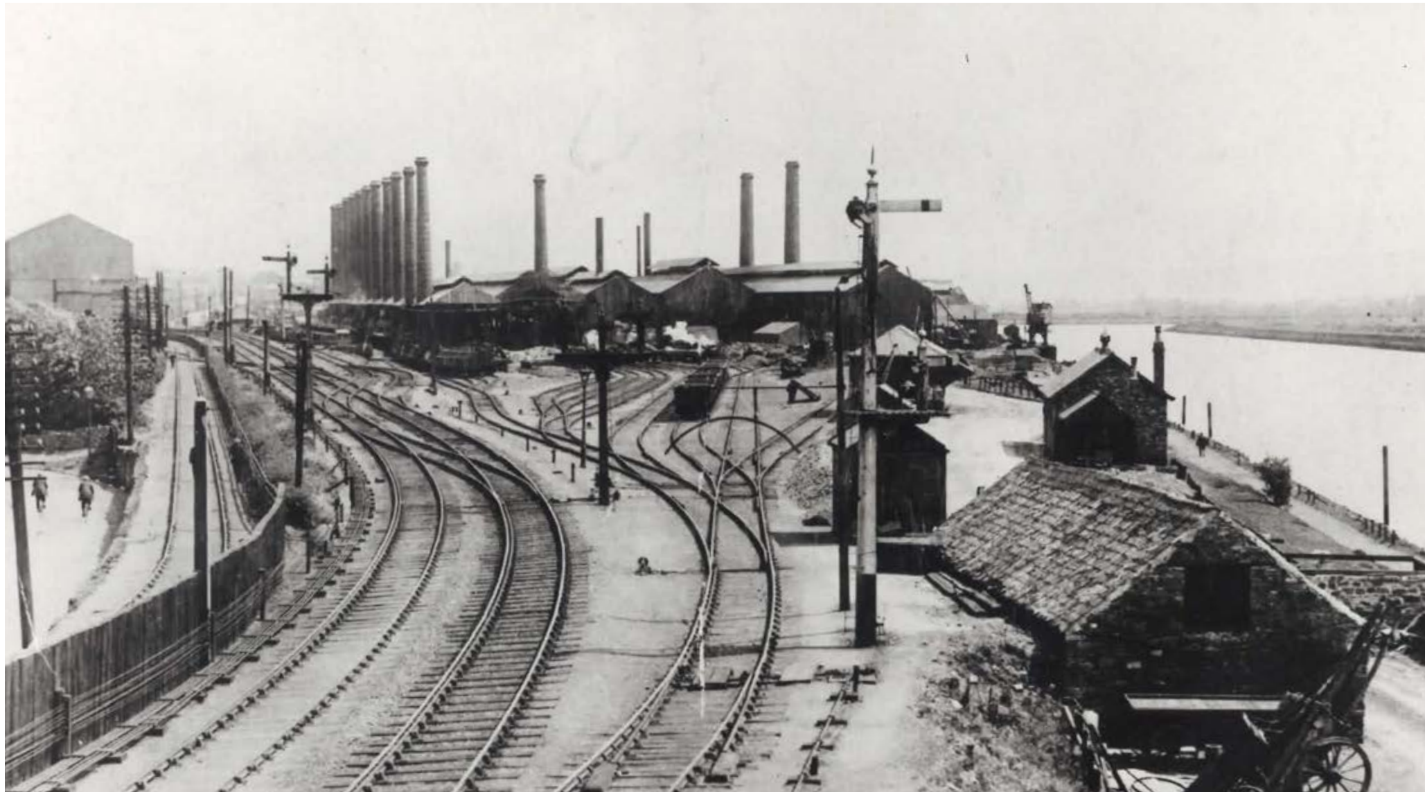
Spencer's Steelworks: In 1811 John Spencer set up a steelworks in the dene to the north of Newburn. The 19th century was a period of rapid industrial development on Tyneside, and demand for the company's products boomed. Spencer's soon became one of the most advanced steel producers in the country. The works expanded until the site spread all the way south to the river. It had its own railway system, including a line to transport coke from Isabella Pit on the other side of Newburn.
